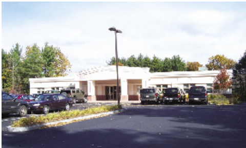
755 Banfield Road - Portsmouth, NH
