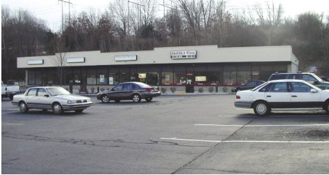
265-297 Providence Street - West Warwick, RI
