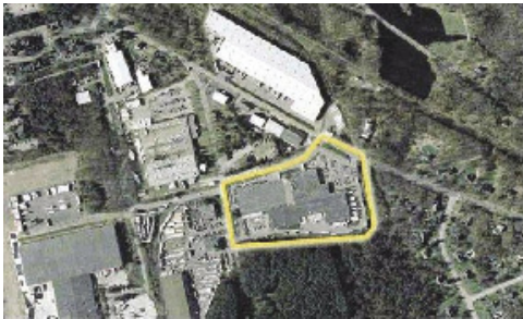
Aerial, 60 Maple Street - Mansfield, MA
