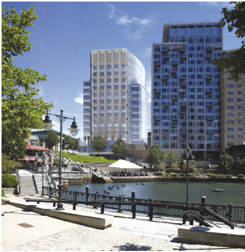
Construction of headquarters for BCBSRI
