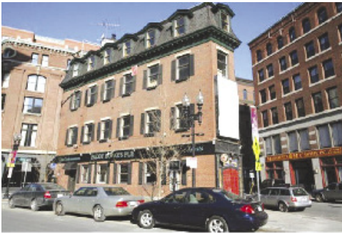
126-132 Portland Street - Boston, MA
