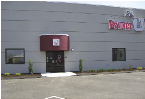
305 Hathaway Drive - Stratford, CT
