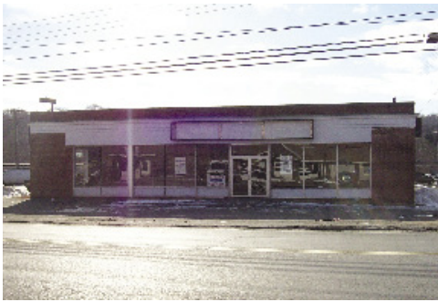
67 Thomaston Avenue - Waterbury, CT
