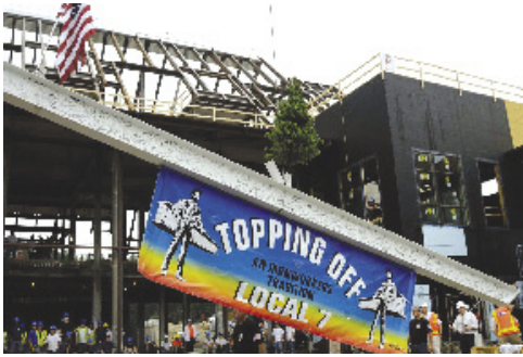
Topping off on NewBridge on the Charles
