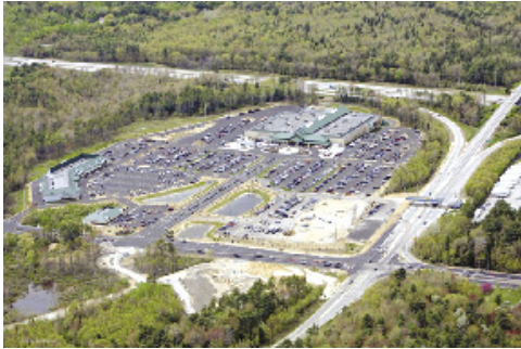
Aerial, Gateway at Scarborough
