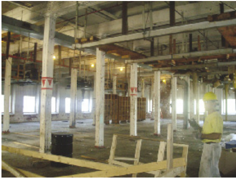
Construction on The Monadnock Mills
