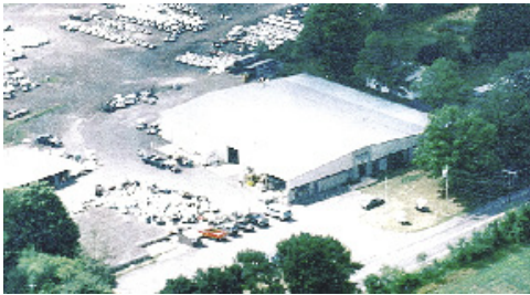
25 West Street - Bolton, CT
