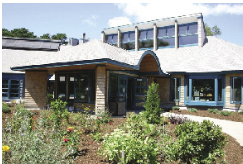
Exterior, Wellfleet Bay Wildlife Sanctuary
