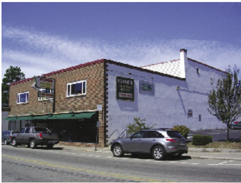
51 Islington Street - Portsmouth, NH
