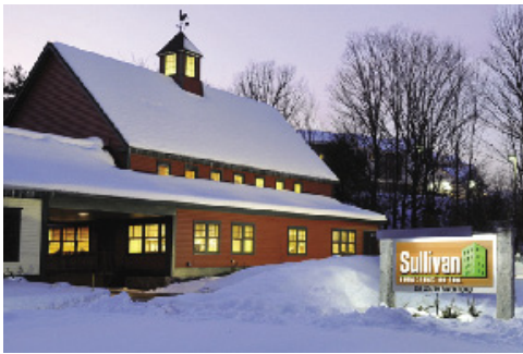
258-260 South River Road - Bedford, NH
