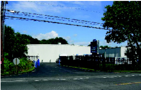
Eastern Bank's self storage facility
