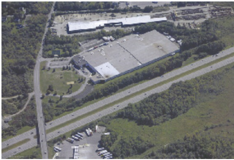
Aerial, 150 Ocean Road - Greenland, NH
