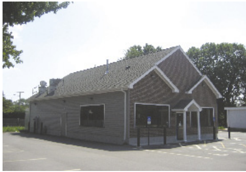
430 Newport Avenue - East Providence, RI
