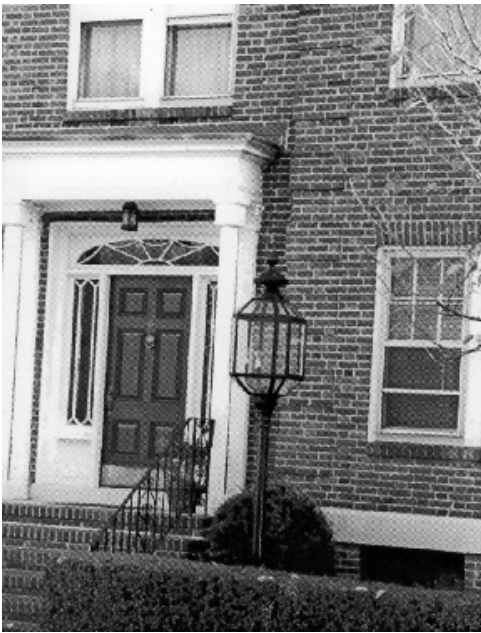
4-26 Alton Court - Brookline, MA, a condo conversion of seven 3-family buildings
