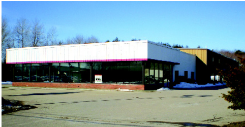
3612 Lafayette Road - Portsmouth, NH
