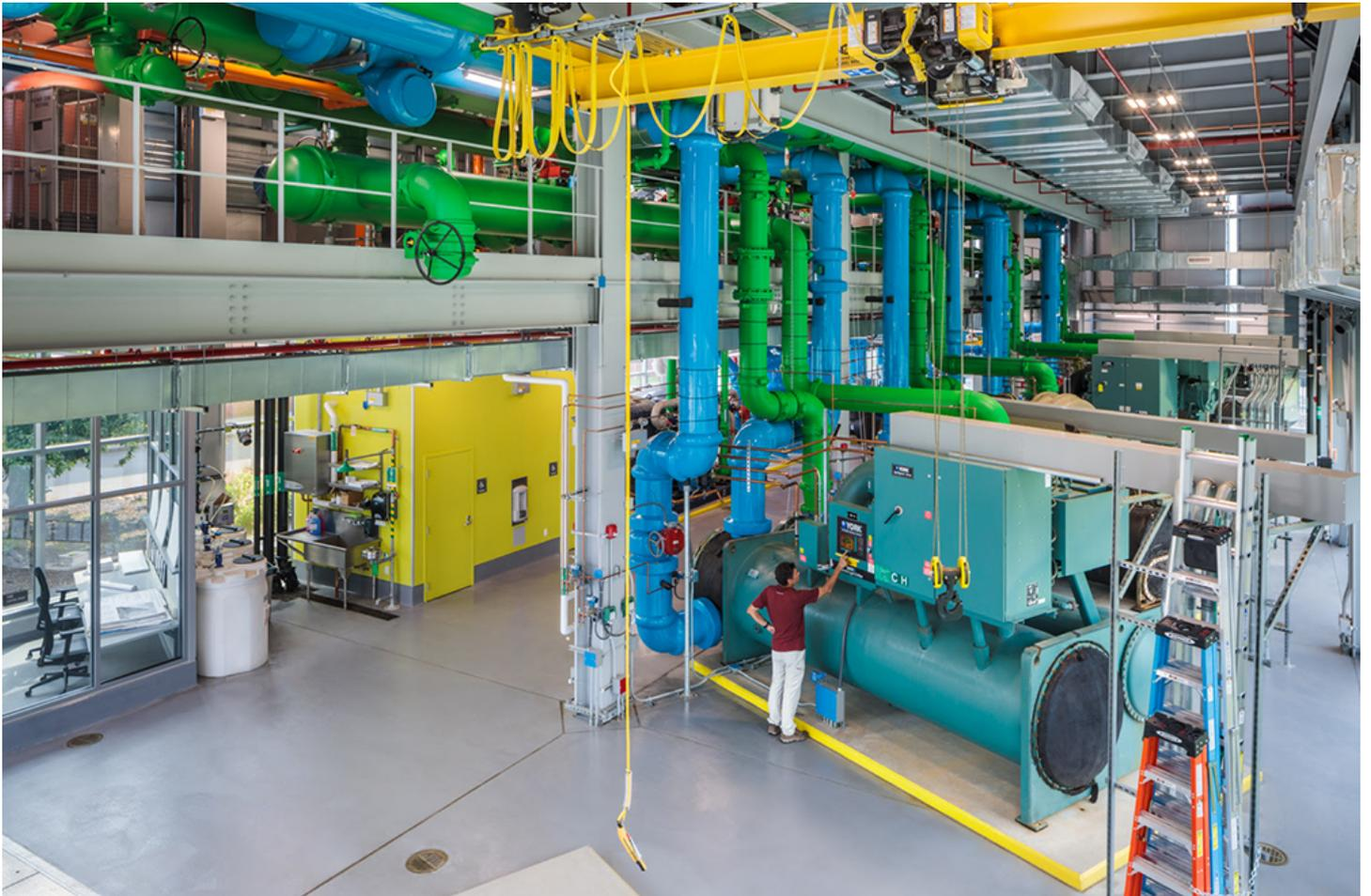
Amherst, MA Leers Weinzapfel Associates' new 10,592 s/f chiller plant at the University of Massachusetts Amherst is the latest in the firm's extensive portfolio of infrastructure work. A component of the university's 2012 Campus Master Plan, it will increase the reliability and capacity of chilled water service throughout its growing north campus core by re-imagining the existing regional plant it replaces.
