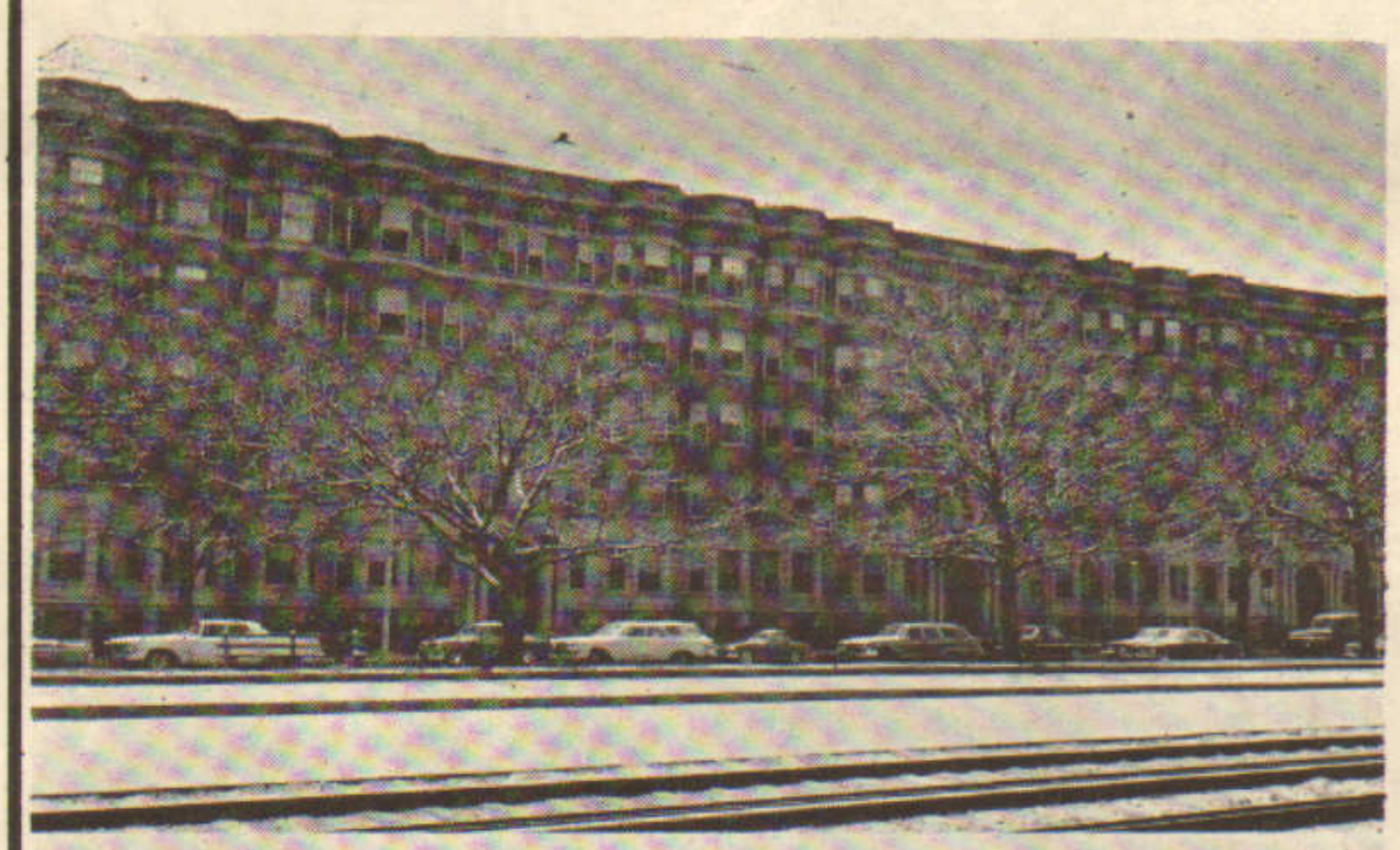
1148-1152-1156-1160 COMMONWEALTH AVE., BOSTON
