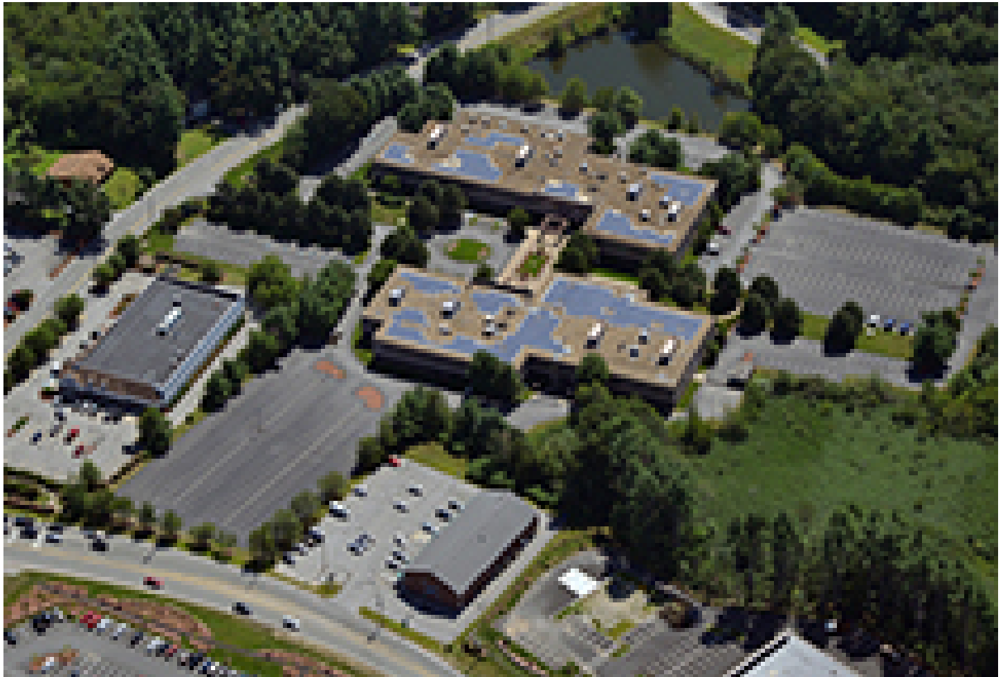
3 & 5 Carlisle Road - Westford, MA
