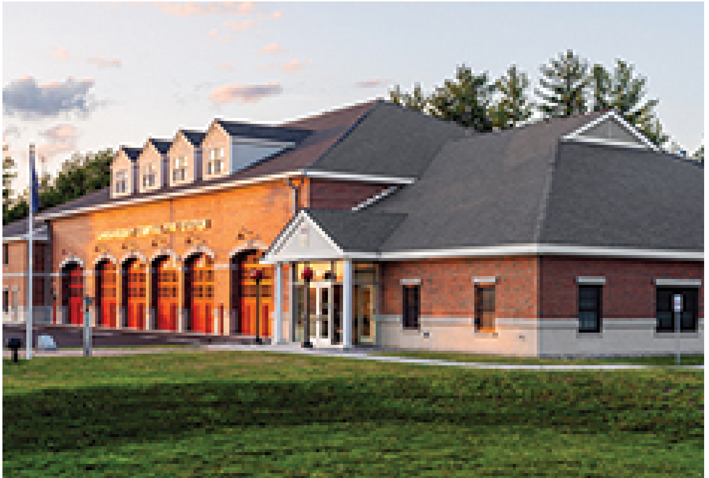
Londonderry Central Fire Station at 280 Mammoth Road - Londonderry, NH
