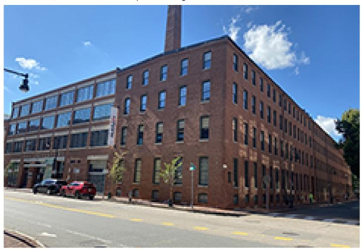
Cambridge, MA Abbot Building Restoration is nearing completion of a masonry repair and waterproofing project involving 14 interconnected four-story occupied office buildings located at 25 First St. in the Kendall Sq. section of the city. The buildings consist of solid, multi-wythe brick exterior walls with precast and granite windowsills and steel lintels.
