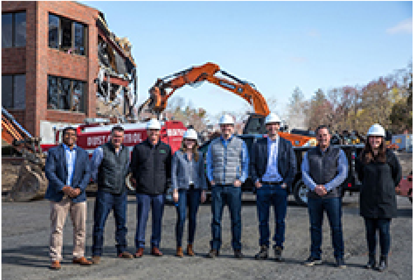
Revolution Labs team from Greatland Realty, Callahan Construction, JLL and SGA at ground-breaking. Photo credit: Nate Photography
