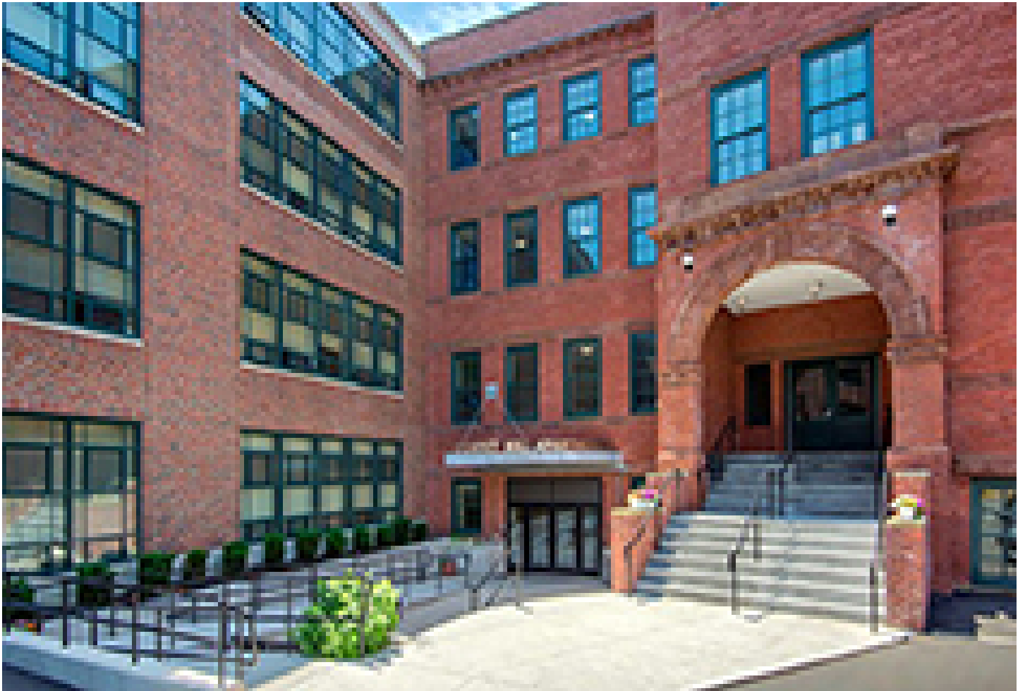
Lofts at Cargill Falls Mill - Putnam, CT
