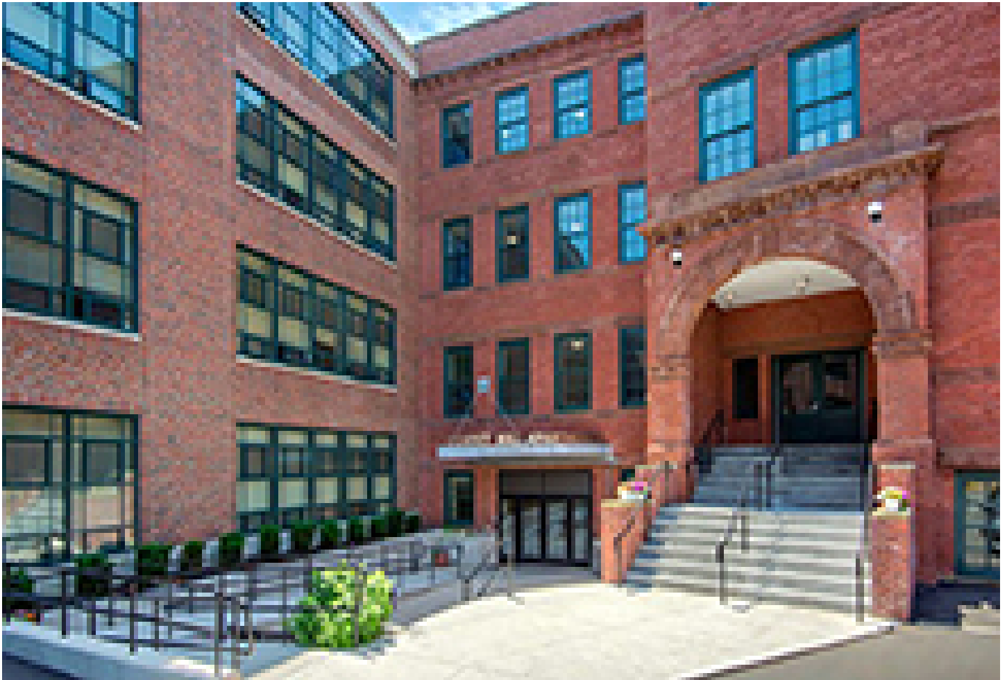
Lofts at Cargill Falls Mill - Putnam, CT
