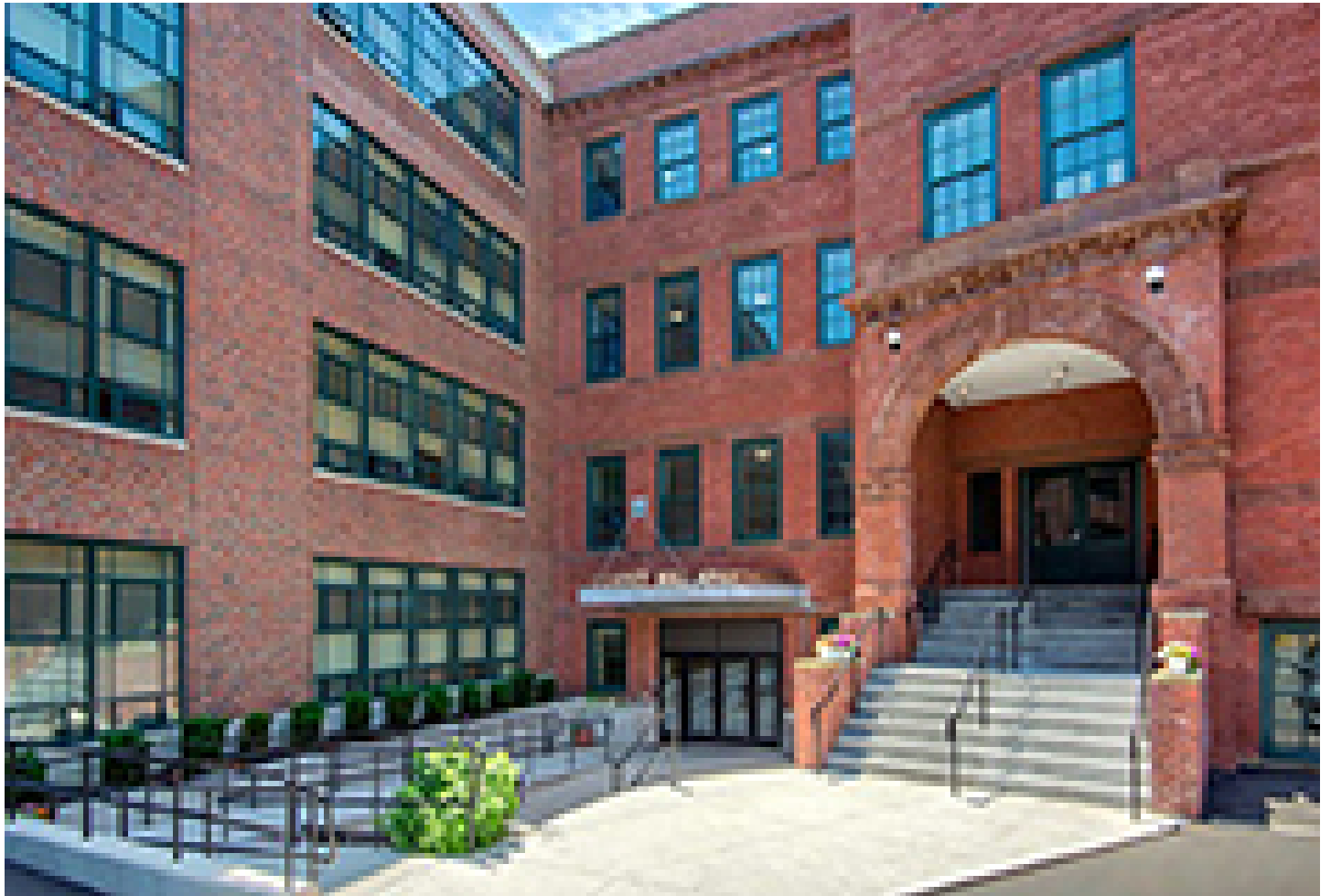
Lofts at Cargill Falls Mill - Putnam, CT
