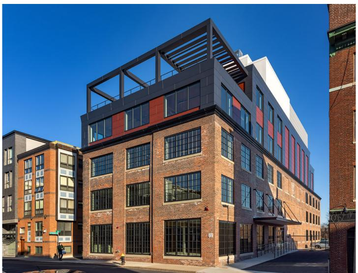
South Boston, MA Margulies Perruzzi (MP) has completed renovations and a two-story addition at 69 A St., creating a five-story 45,000 s/f building that is the first "cross-laminated timber" (CLT) addition to an existing building in downtown Boston.
