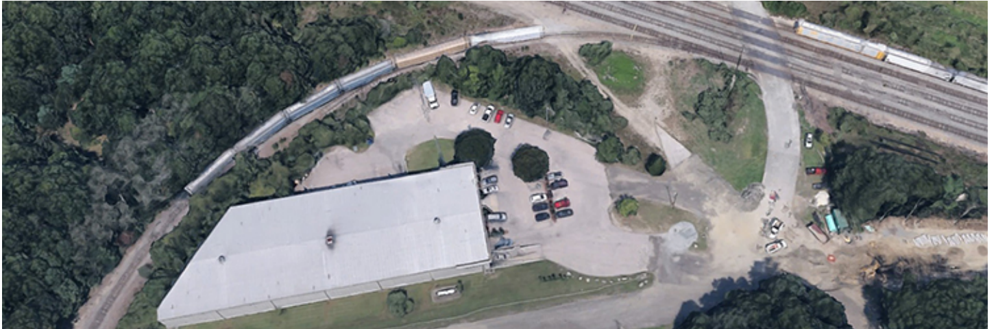
Aerial View of 135 Compass Circle - Quonset Business Park - North Kingstown, RI
