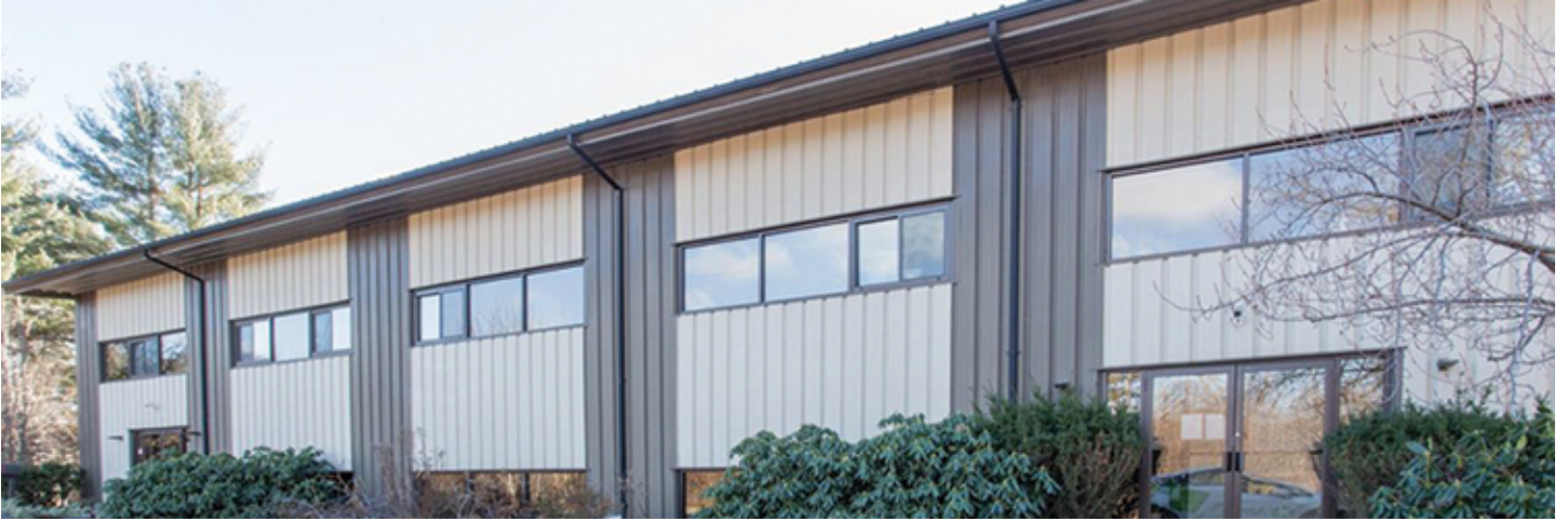
Caption 200 Turnpike Road - Southboro MA
