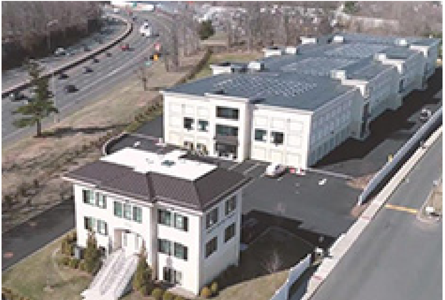
Hollow Tree Self Storage - 131 Hollow Tree Ridge Road - Darien, CT
