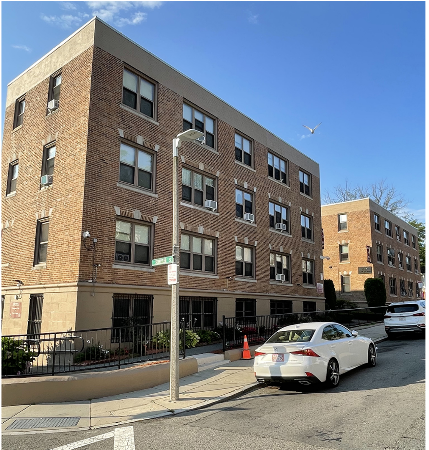
Dorchester, MA Abbot Building Restoration Company, Inc. completed a comprehensive masonry
