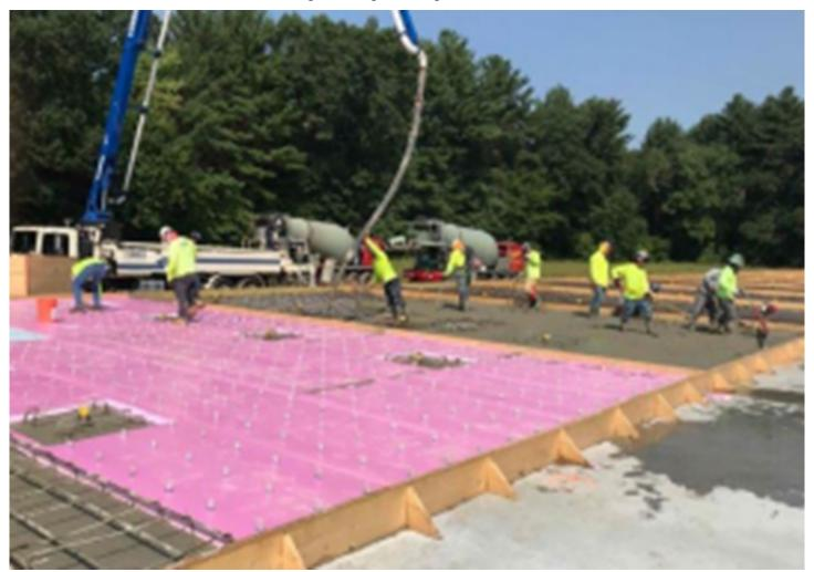
Norton, MA According to Condyne Capital Partners and Polar Design Build, the tilt up walls are ready for install at Home Depot warehouse. All site work has been completed including the laying of utilities, foundation poured, and ground has been leveled. The tilt up panels have been framed, insulated, cured, and are now ready for installation.
