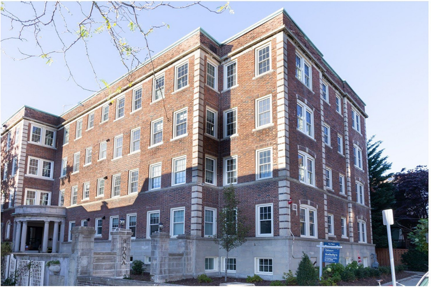
Cambridge, MA South Coast Improvement Company (SCIC), a design-build general contractor, has completed work on a $6.75 million renovation project for Rafi Properties at 9 Dana St. The Marion,
