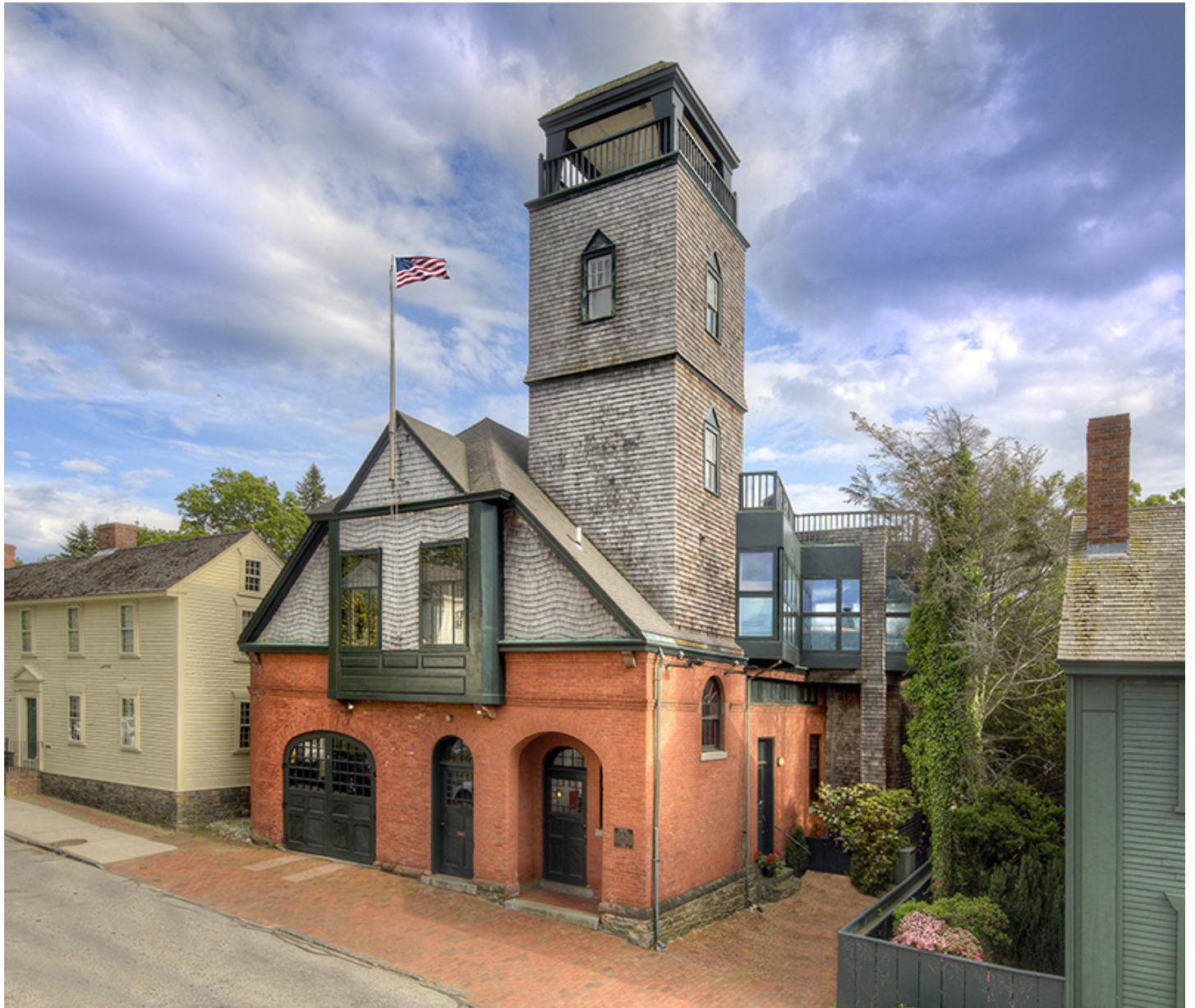
Fire Station No. 1, 25 Mill Street - Newport, RI
