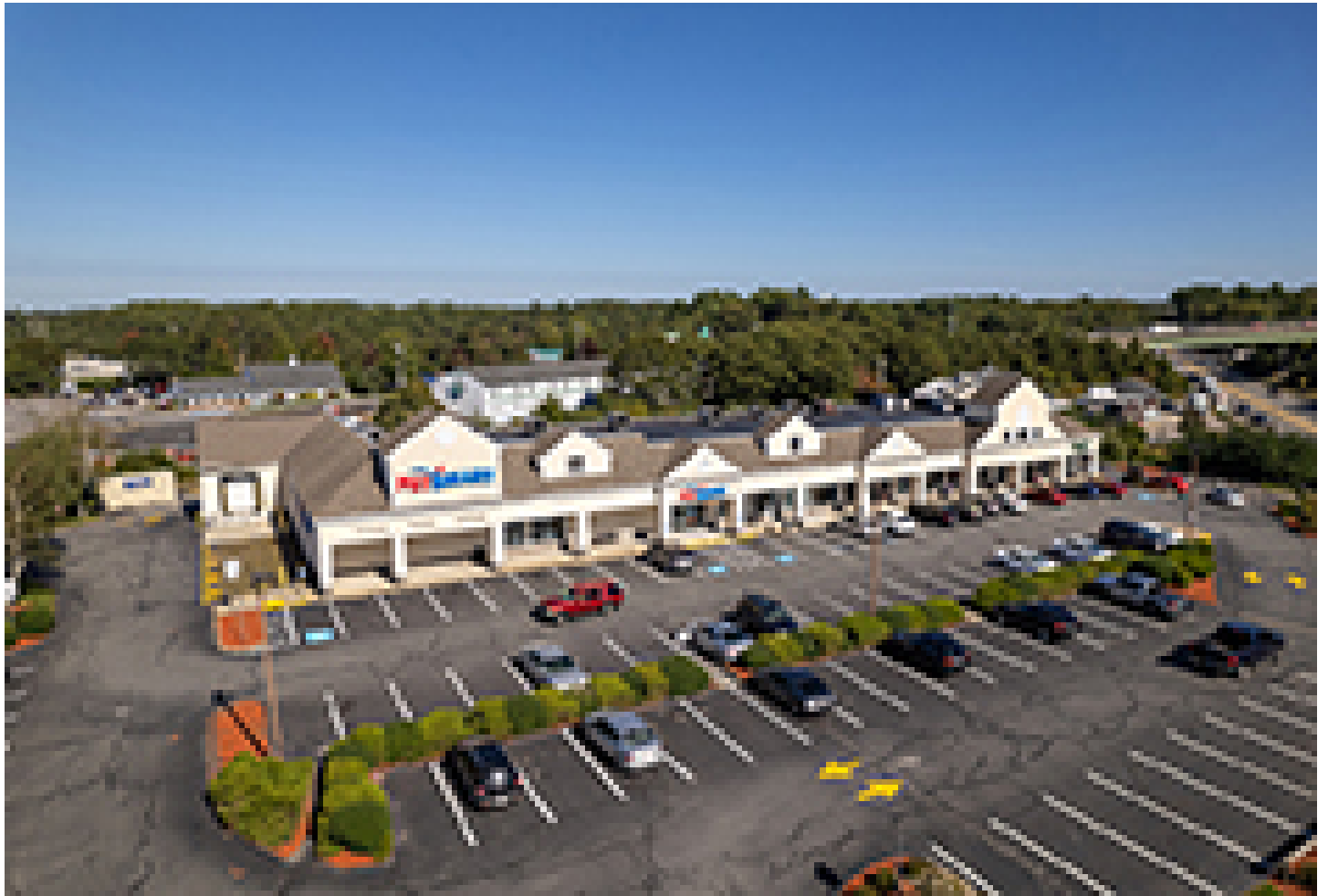
Bourne Bridge Crossing, 2 Bridge Approach Street - Bourne, MA
