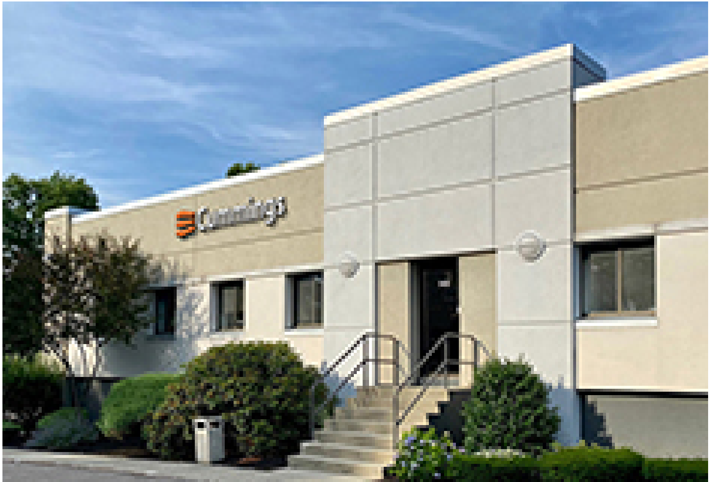
50 Tower Office Park - Woburn, MA
