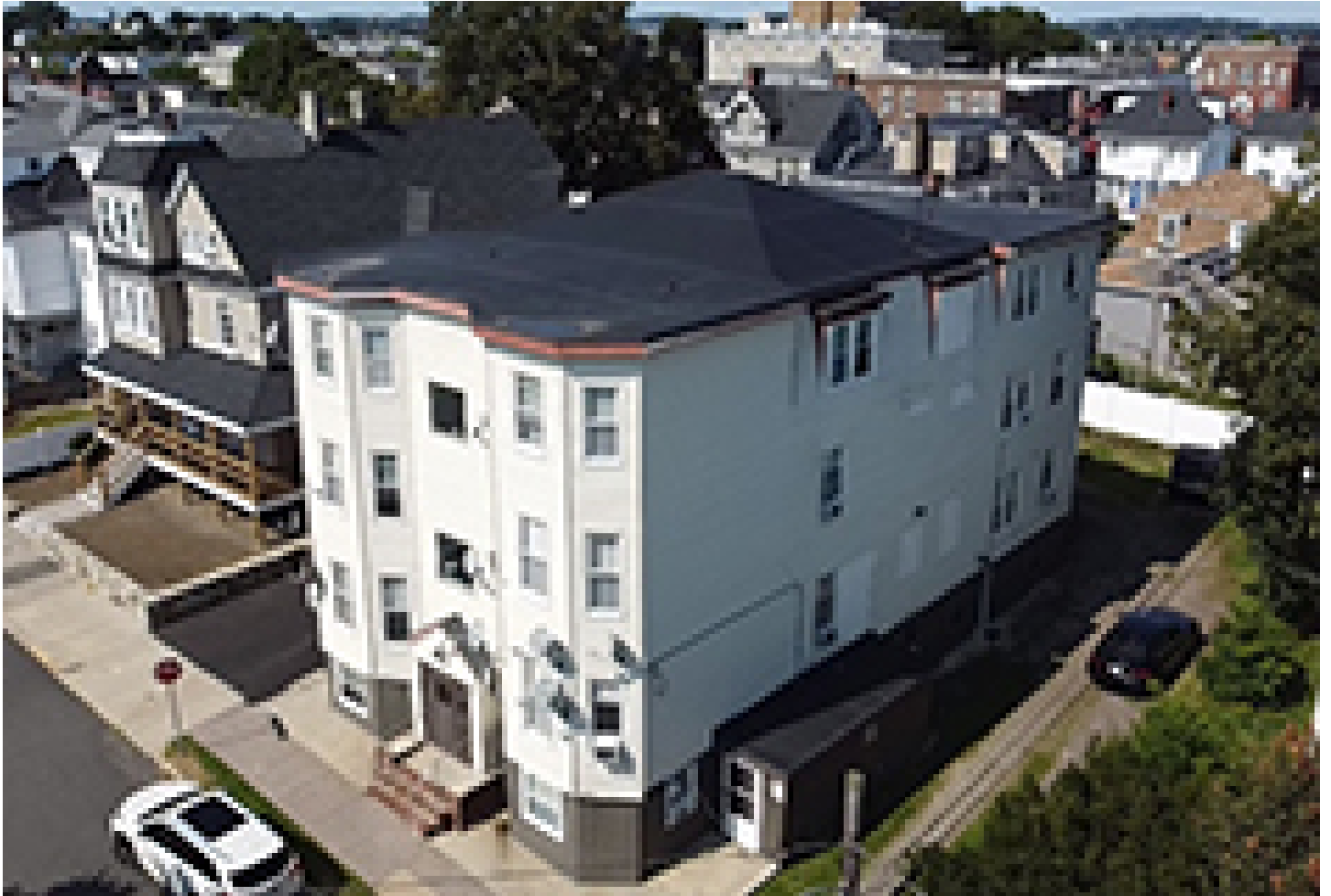
Fitzhenry Square Apartments - Revere, MA
