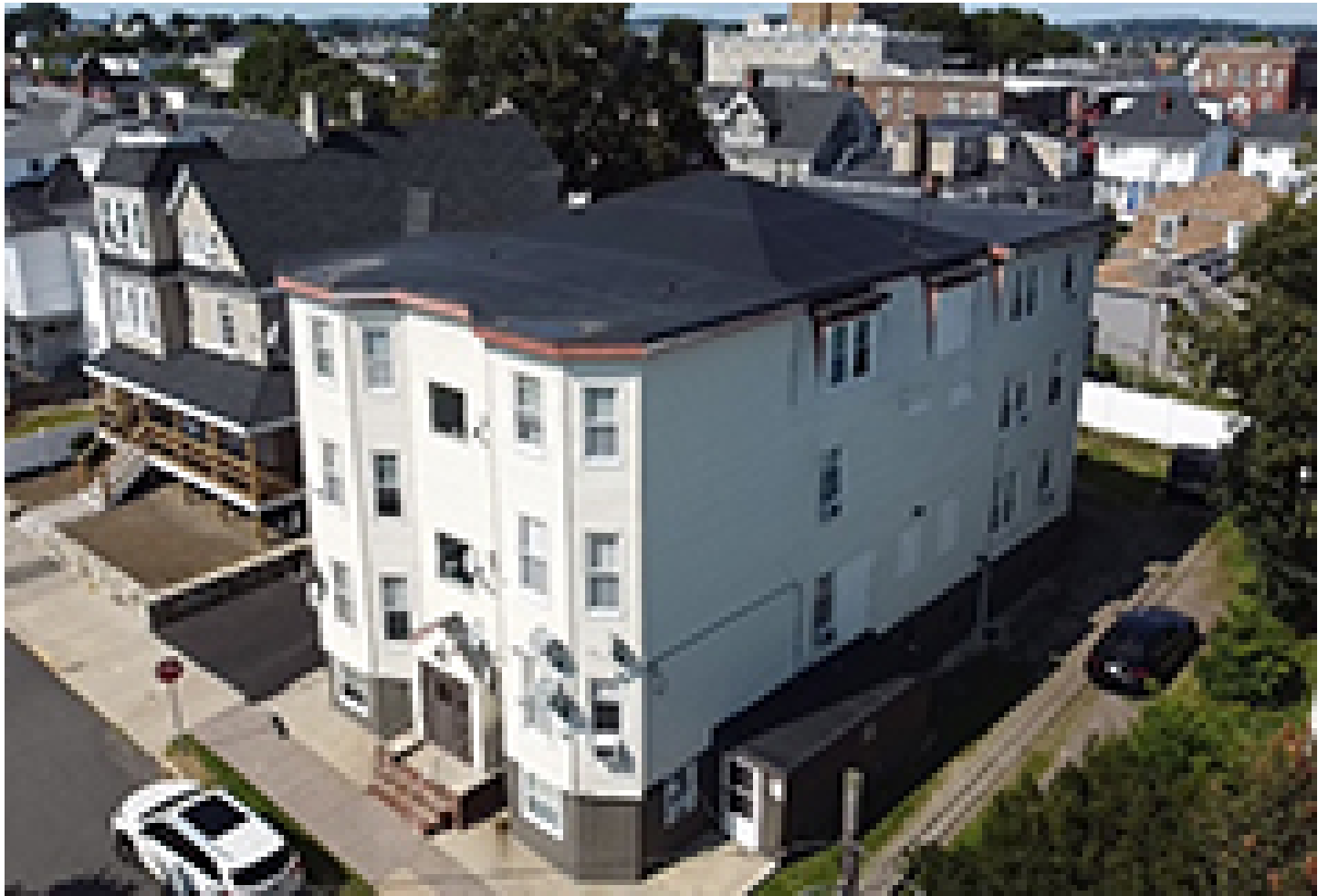
Fitzhenry Square Apartments - Revere, MA
