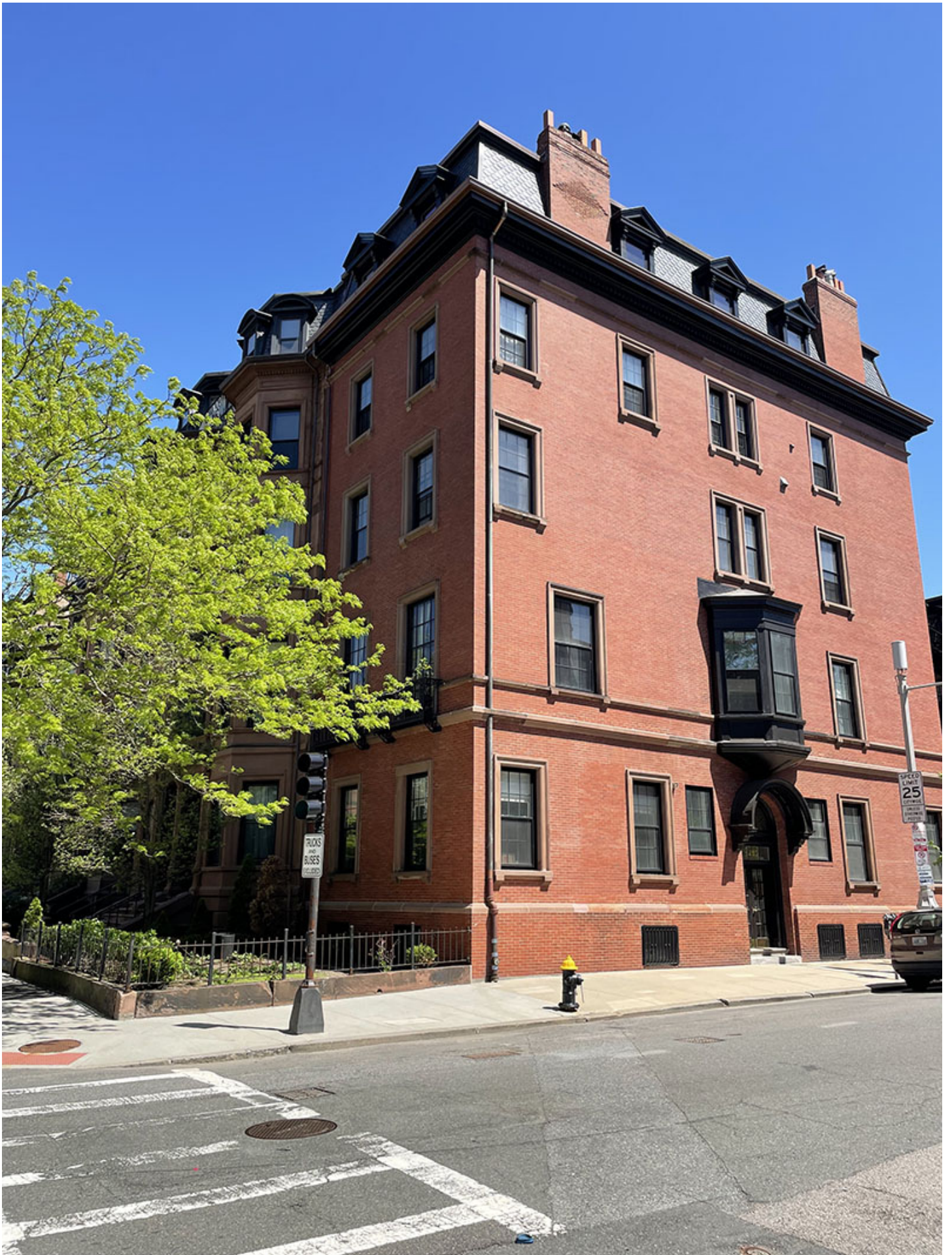
Boston, MA Abbot Building Restoration Company, Inc., recently completed a major masonry restoration and replacement project on a five-story brownstone and brick condominium building
