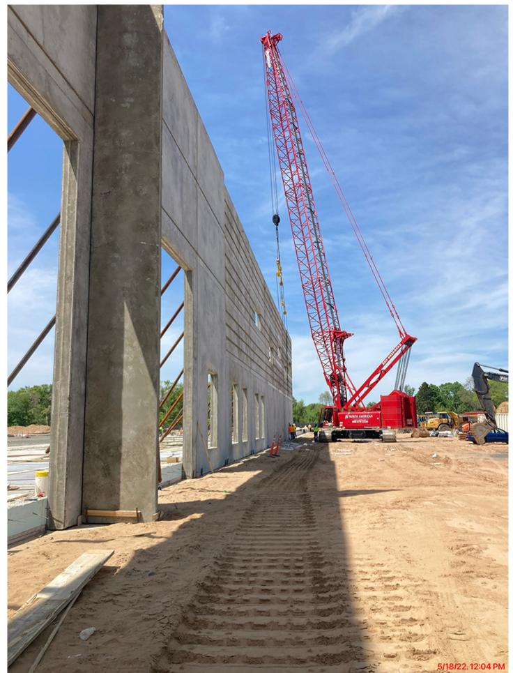
Windsor, CT According to Condyne Capital Partners and Polar Design Build tilt-up walls have been fabricated and erected for the Baker Hollow Logistics Center. All site work has been completed
