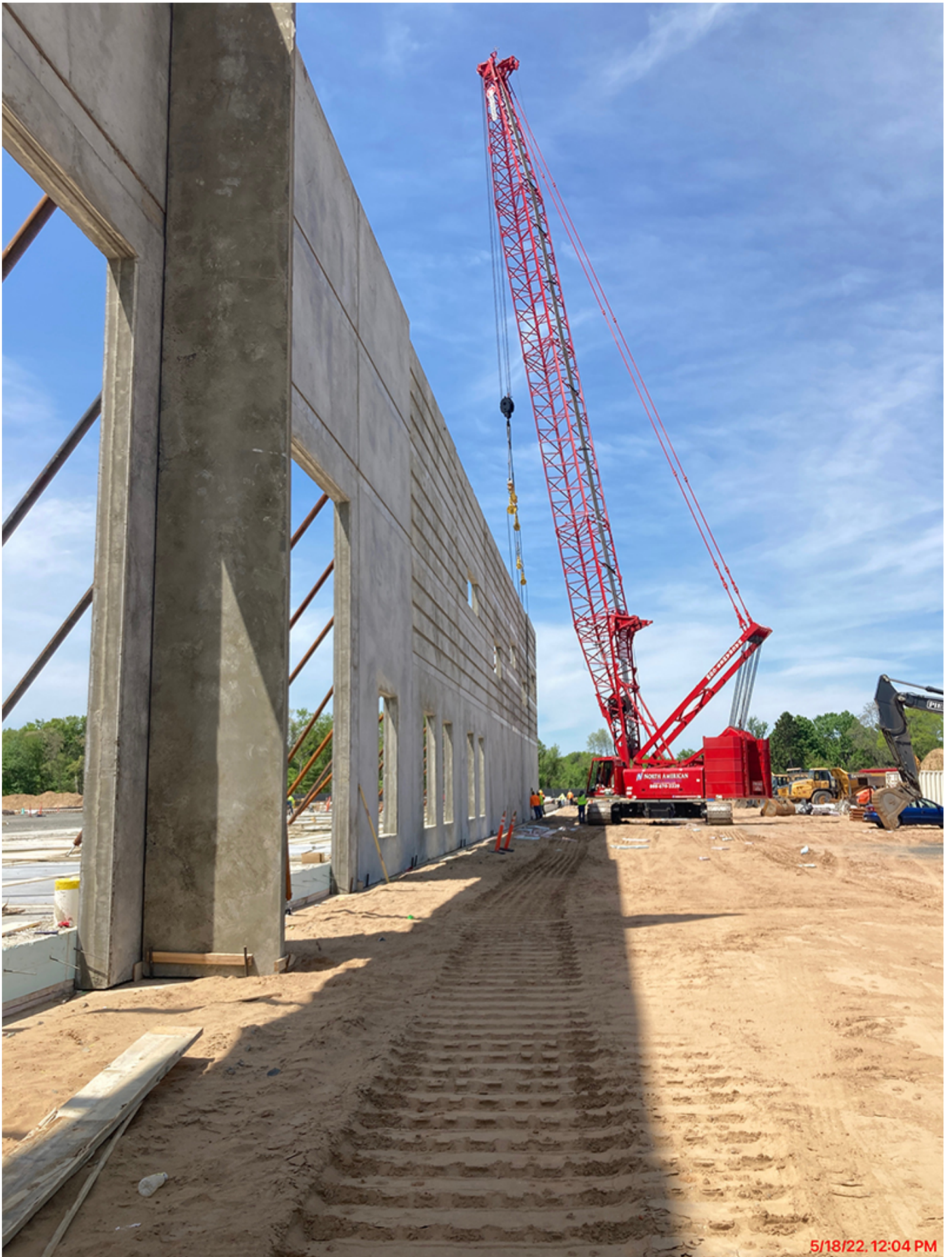
Windsor, CT According to Condyne Capital Partners and Polar Design Build tilt-up walls have been fabricated and erected for the Baker Hollow Logistics Center. All site work has been completed
