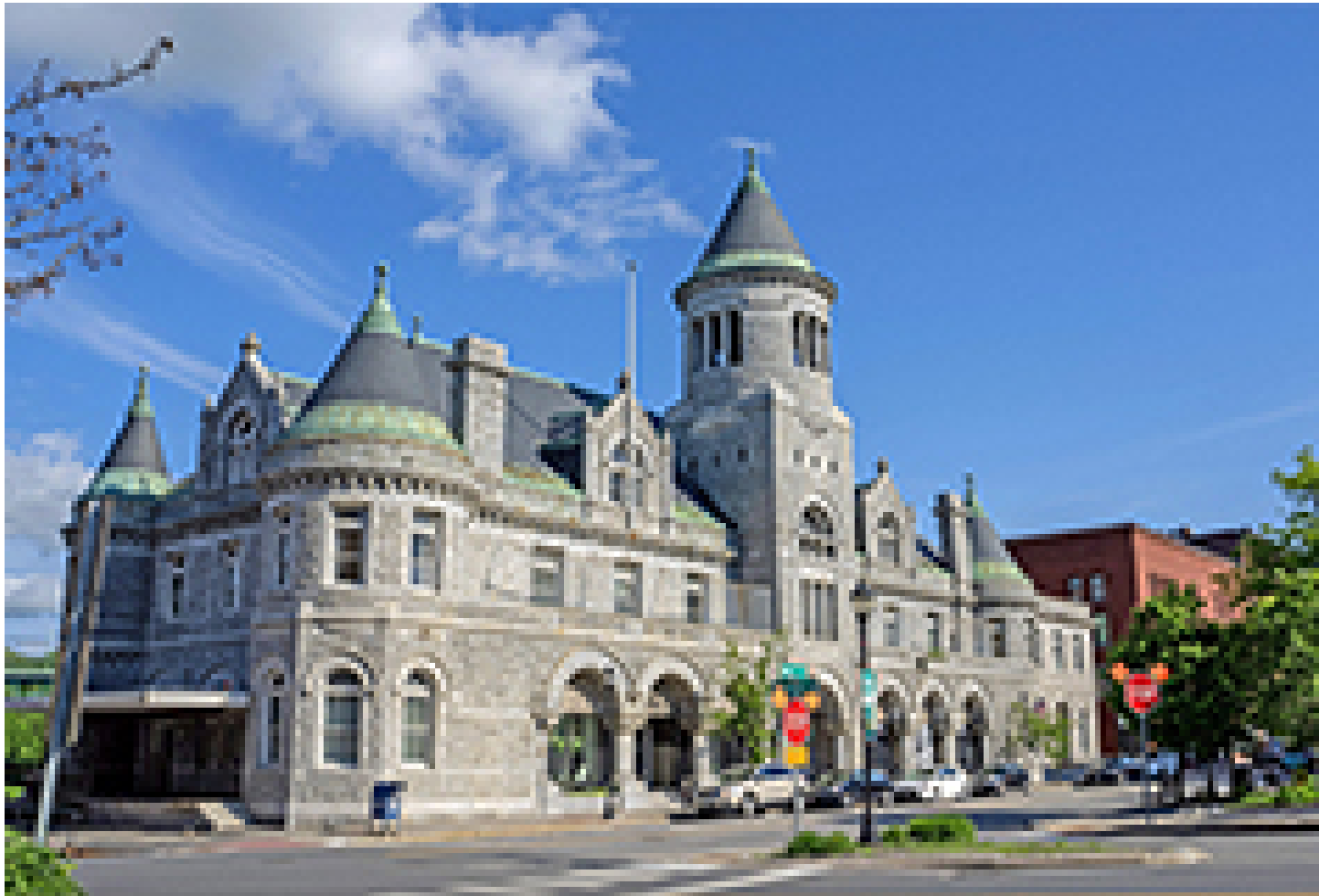
Olde Federal Building, 295 Water Street - Augusta, ME
