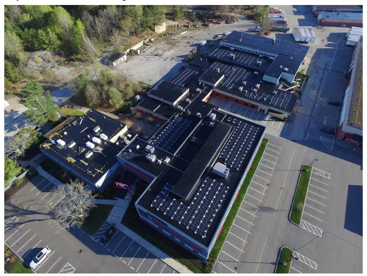
Hooksett, NH PROCON has completed a 139-kilowatt solar array that sits atop the company's headquarters. The array will generate an estimated 154,377-kilowatt (kW) hours of renewable energy each year, offsetting nearly 50% of the company's electric load and over 151,000 pounds of annual carbon emissions.
