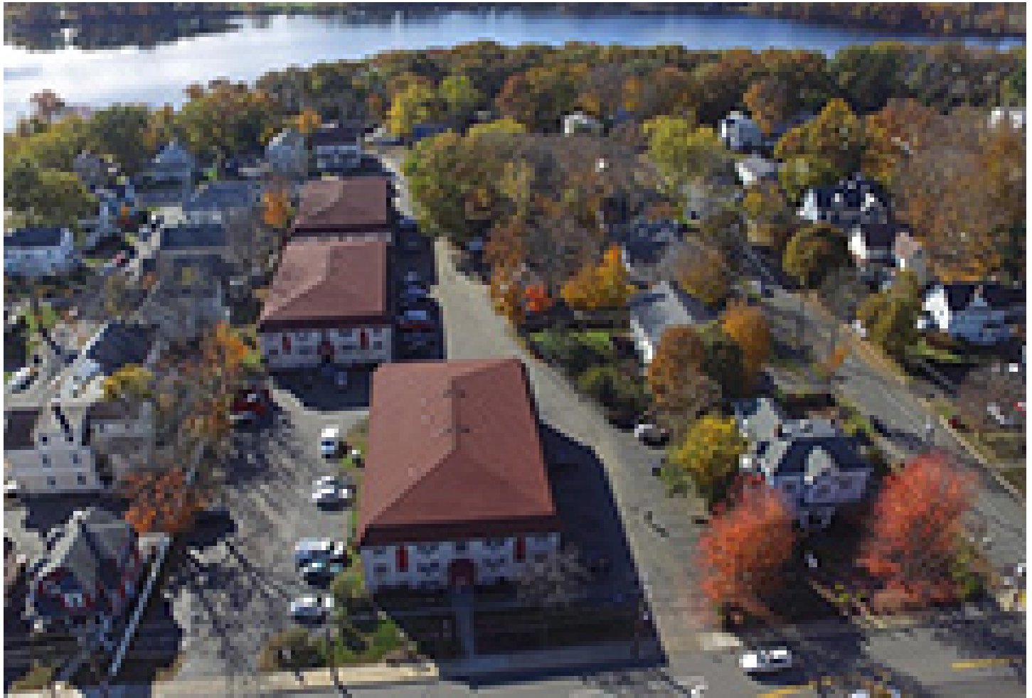
258 Union Avenue, Rose Garden Apartments - Framingham, Mass.
