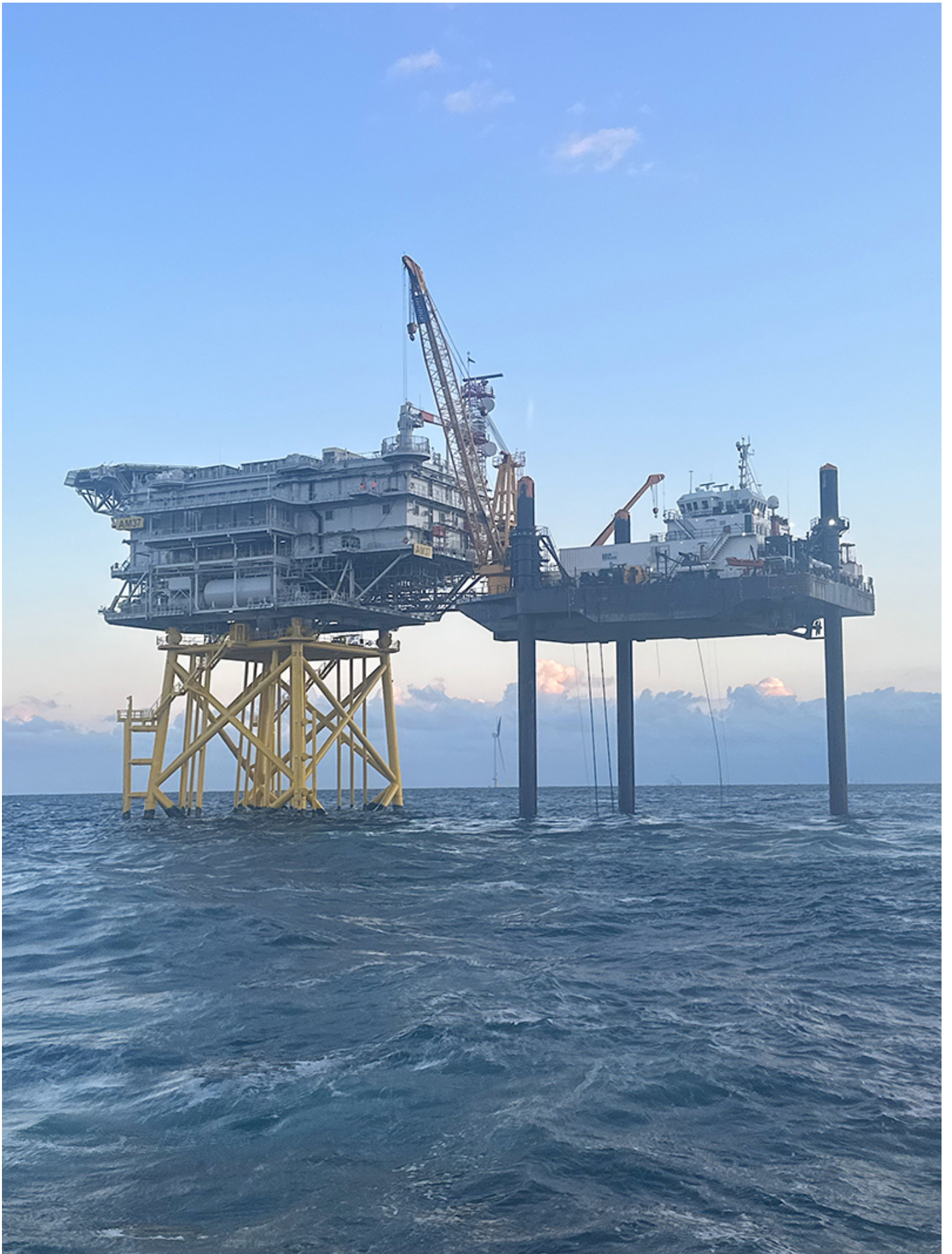
The Vineyard Wind 1 Electrical Service Platform (ESP)
