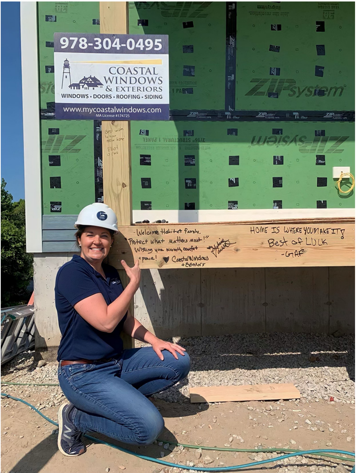
Concord, MA Supporting Habitat for Humanity of Greater Lowell's housing program during Women in Construction Week, Coastal Windows & Exteriors (CWE) attended the 52nd Home Dedication
