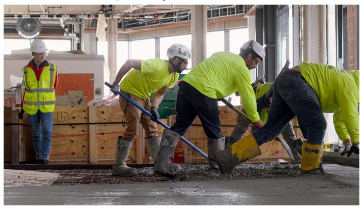
Boston, MA WS Development and Sublime Systems have completed the first-ever commercial application of low-carbon Sublime Cement, manufactured by Sublime Systems, which spun out of MIT in 2020. The concrete placement is located in the indoor public space of WS Development's One Boston Wharf, one of the city's largest net-zero-carbon office buildings, in the Seaport district.
