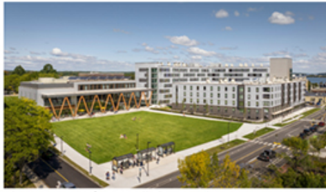
Photo courtesy of Trent Bell Photography
