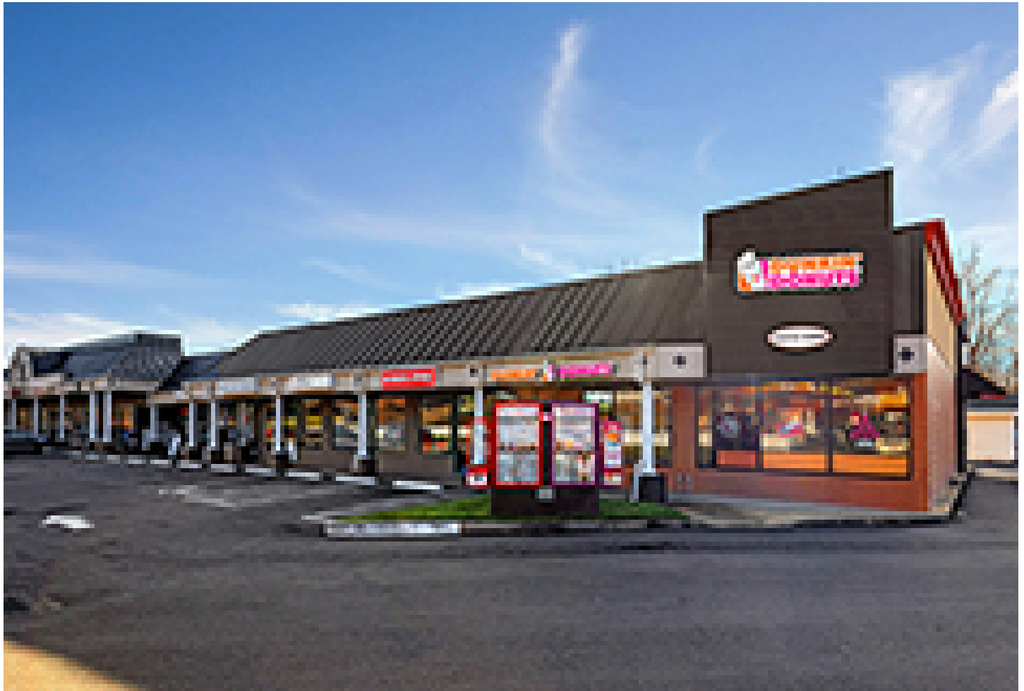
Salem Plaza at 1 New London Road - Salem, CT
