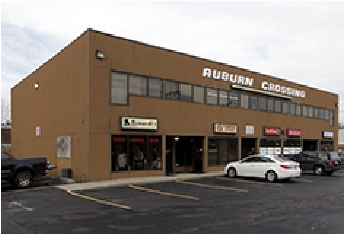
Auburn Crossing Building, 482 Southbridge Street - Auburn, MA
